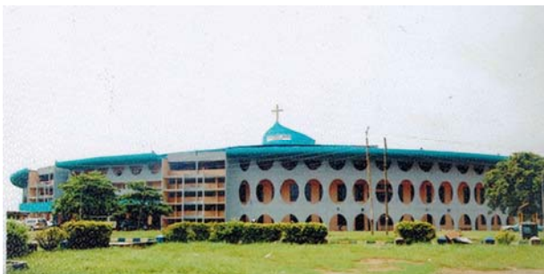
The TACLAWNA Convention Centre—Lagos
